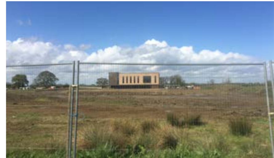
View north across Design Code area towards the existing Whitehouse Health Centre
