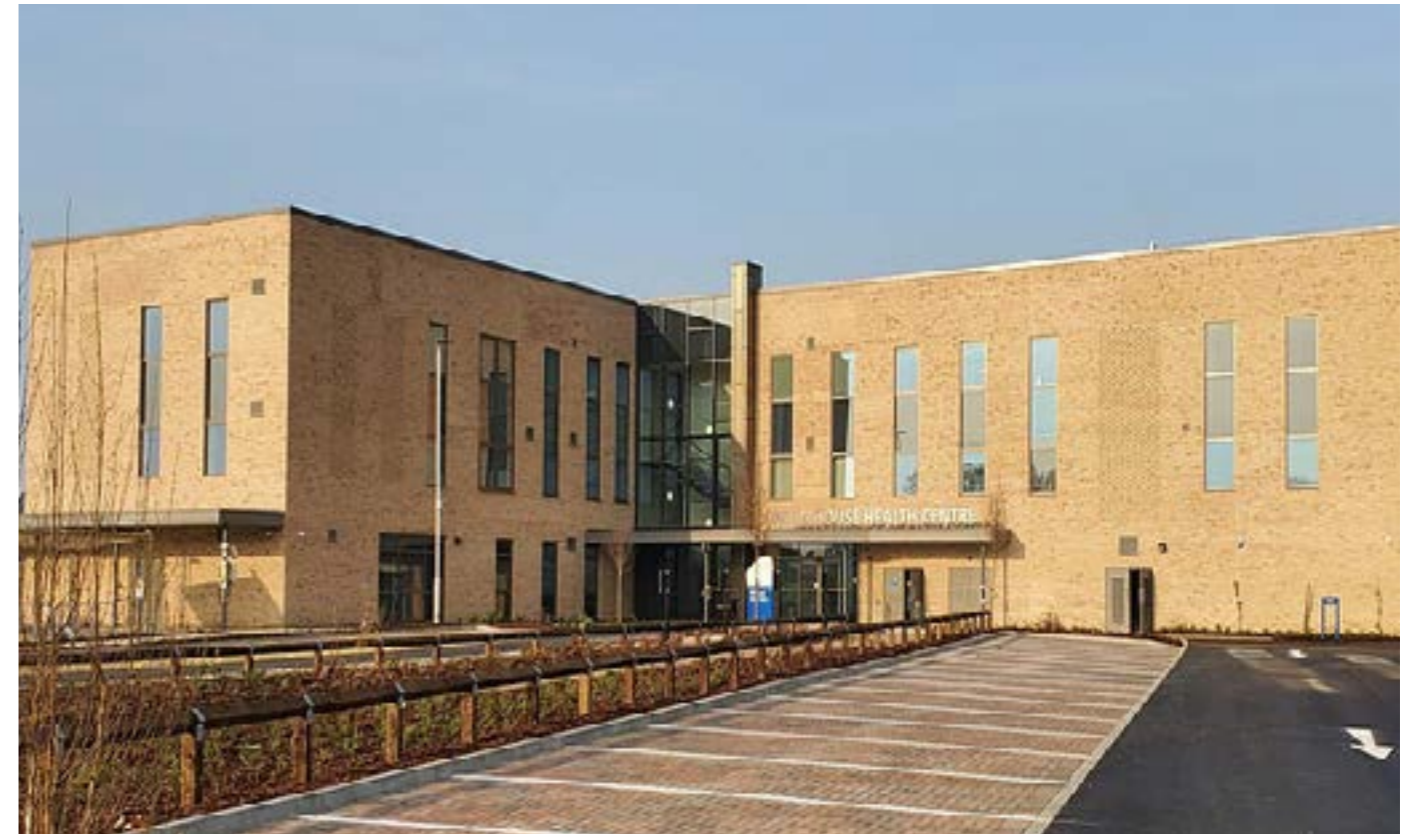
Images of Existing Whitehouse Health Centre
