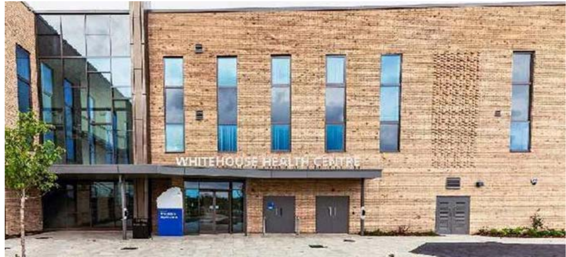
Images of Existing Whitehouse Health Centre
